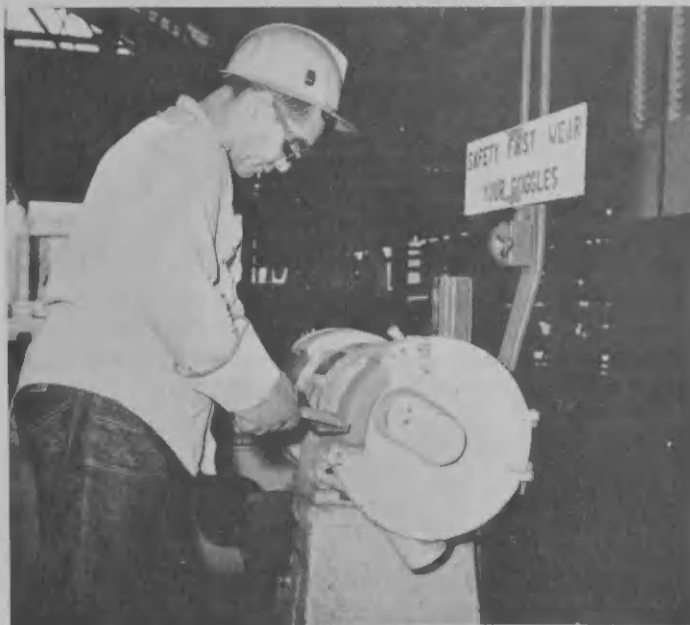
WORK ON grinders requires the use of safety goggles as used by this Mechanical tradesman.
